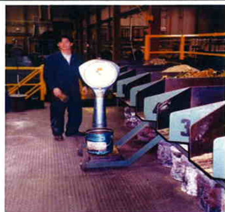
Fig 6 Storage Hoppers and weighing Station of Furnace Platform
